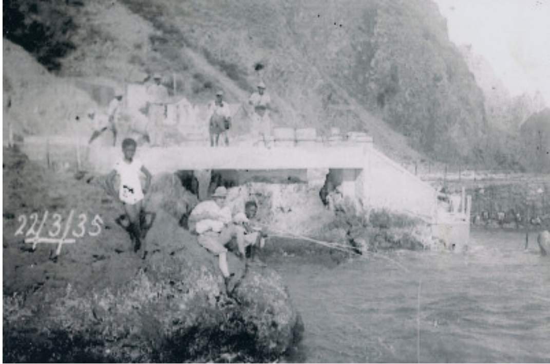
Old pier at Fort being built with Mr. L.B.Scott standing on the pier. Photo by Steve Kruythoff 1935
